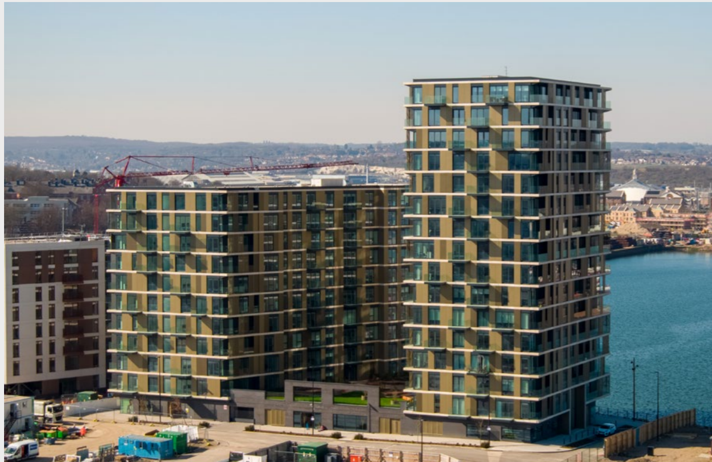
Drone image of the completed two towers of X1 Chatham Waters
